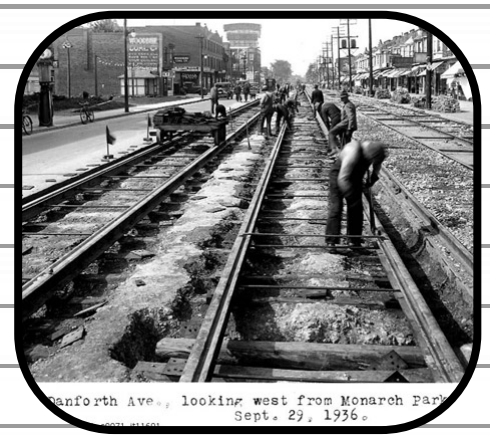
Streetcar construction on Danforth Ave, 1936
